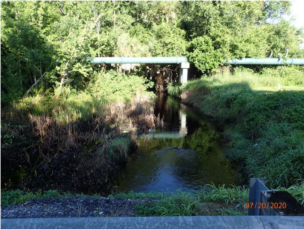
Channel Looking West
